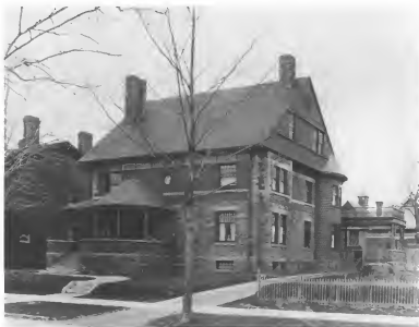
View of the Metcalfe house, 125 North Street, Buffalo, soon after it was completed in 1884. The house was demolished in 1980.
